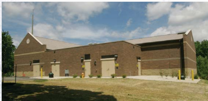
Well 5 - Pelham Road
