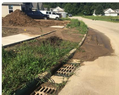
Silt fence was never installed and therefore sediment is leaving the site.
