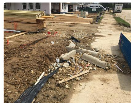
Silt fence was installed improperly and never maintained. Construction debris knocked the silt fence over and sediment is leaving the site.
