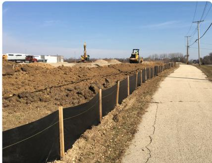
The silt fence is properly installed meaning it is trenched and back filled.
