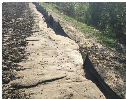
The silt fence is properly installed but needs maintenance. Once sediment is half way up the silt fence the sediment needs to be removed and the silt fence needs to be repaired.
