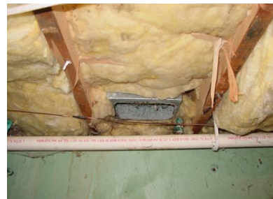
Figure 2151-3: Combustion air intake from crawl space; floor above crawl space is thermal boundary
