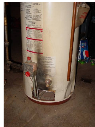
Figure 31111-1: Evidence of flame roll-out
