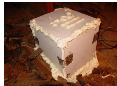
Figure 2131-1: Recessed light covered with drywall box
