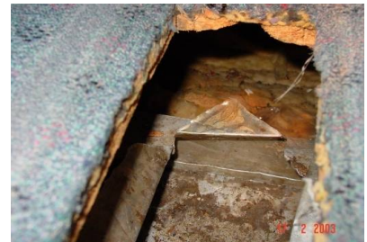
Figure 4114-1: Opening between duct boot and floor
