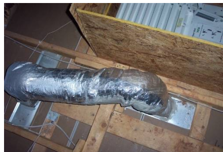
Figure 1153-1: Jumper duct installed in attic connecting bedroom to hallway (Courtesy Southface Institute)
