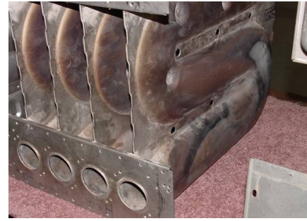
Figure 3151-1: Furnace heat exchanger
