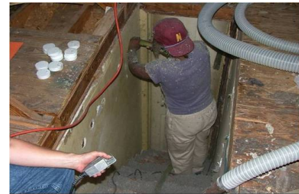
Figure 2135-3: Stairwell walls being dense-packed
