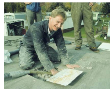
Figure 41612-1: Blowing insulation through mobile home roof
