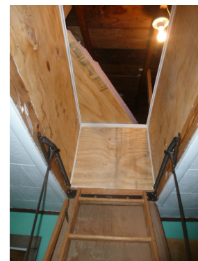
Figure 2135-2: Box around retractable attic stairs
