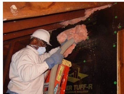
Figure 21364-3: Knee walls being dense-packed with cellulose
