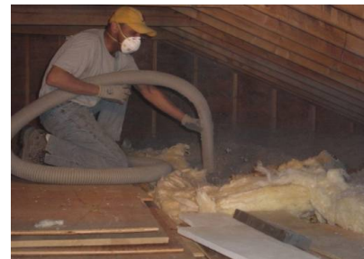
Figure 21331-1: Required attic insulation R-value is a minimum of 49 or the maximum amount with an SIR greater than 1.0
