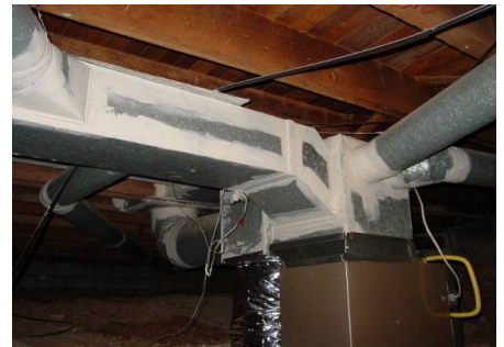
Figure 31532-2: Duct mastic used to seal duct joints
