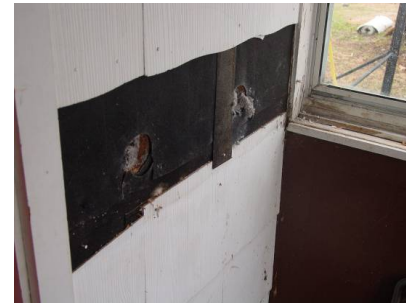
Figure 2141-1: Asbestos siding that has been removed
