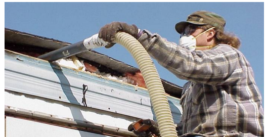
Figure 41611-2: Blowing roof cavity from edge
