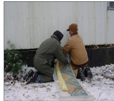
Figure 41521-1: Batt-stuffing a mobile home wall
