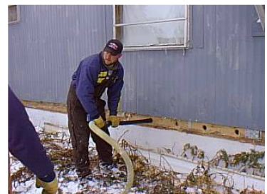
Figure 41421-1: Blowing a mobile home floor from the side
