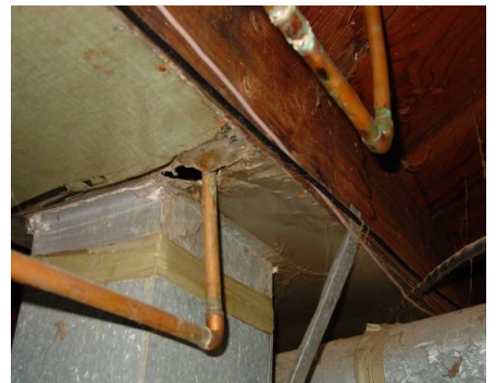
Figure 31531-5: Seal holes in ducts
