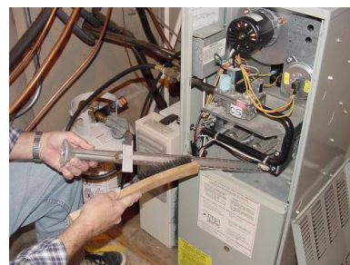
Figure 31111-2: Clean burners with stiff brush
