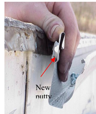
Figure 41611-3: Re-installing roof gutter with new putty tape
