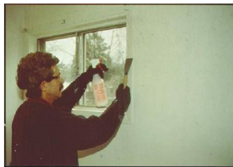
Figure 5132-1: Use hand tools whenever possible
