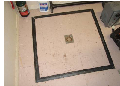
Figure 2153-2: Crawl space access hatch; weatherstripped and easily removable
