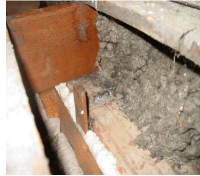
Figure 2122-6: Fur cavity sealed with 2-part spray foam
