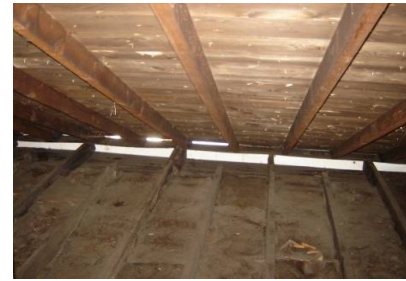
Figure 21324-1: Foam blocking installed over top plates
