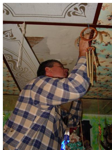
Figure 1111-2: Remove a ceiling tile to relieve pressure
