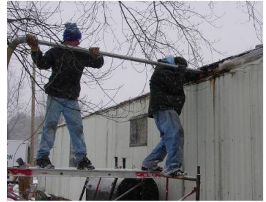
Figure 41611-1: Blowing from the edge
