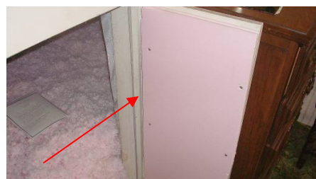
Figure 21365-1: Knee wall hatch insulated and weatherstripped
