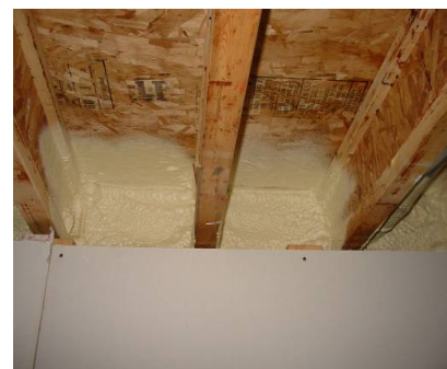
Figure 2171-1: 2-part spray foam on rim joist
