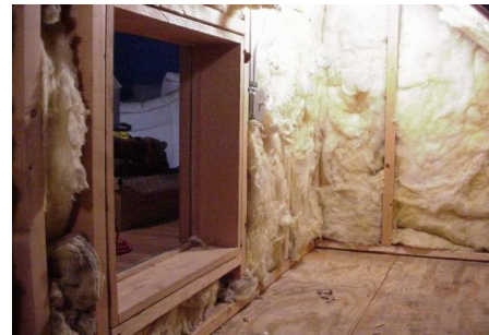
Figure 21364-1: Knee walls insulated with fiberglass insulation
