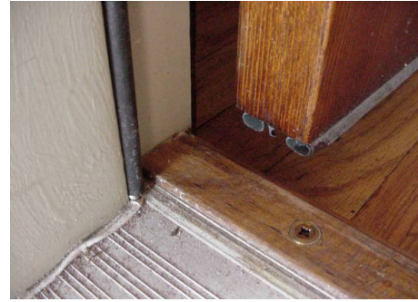
Figure 2191-1: Door weatherstripping, threshold and sweep
