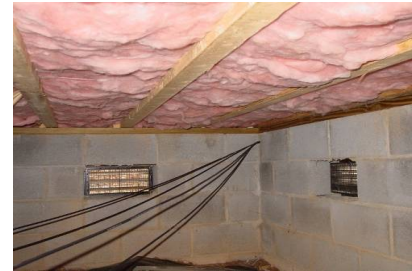
Figure 2152-1: Insulation should fill floor cavity
