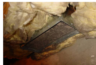
Figure 3113-2: Dirty combustion air intake to wood stove that needs to be cleaned
