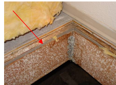
Figure 2153-1: Peel & stick weatherstripping is not permitted
