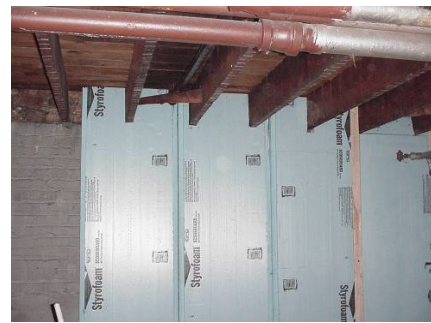
Figure 2161-1: Rigid foam board basement wall insulation
