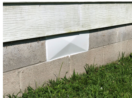
Figure 2155-1: Insulated vent with metal cover.
