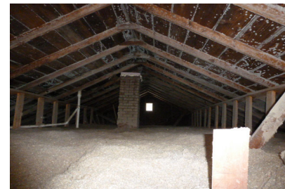
Figure 2122-8: Cut-off chimney in attic
