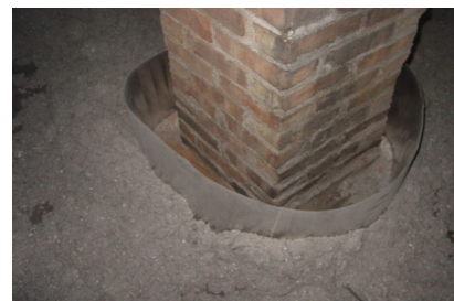
Figure 2131-3: Metal barrier around chimney
