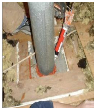
Figure 2131-2: Metal barrier around flue sealed with high temperature caulk
