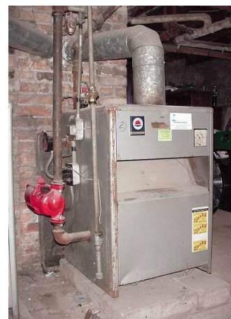
Figure 3161-1: Warm water boiler
