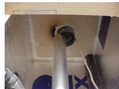
Figure 31111-3: Ensure that vent is properly connected
