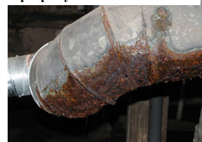
Figure 31111-4: Check vent for condensation problems
