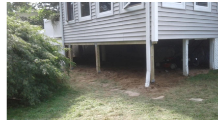
Figure 2154-1: Crawl space supported on piers
