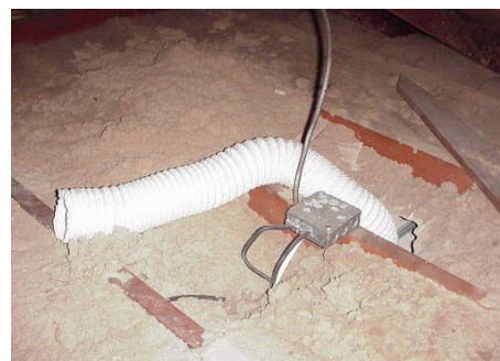
Figure 507-1: Fans may not be vented into the attic under the Weatherization Program
