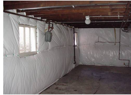
Figure 2162-1: Vinyl faced fiberglass insulation
