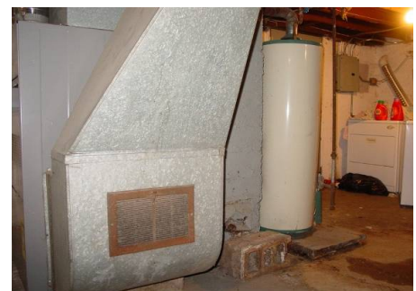
Figure 31531-6: Return air grilles should be sealed
