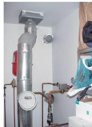
Figure 3124-2: Combustion air intake
