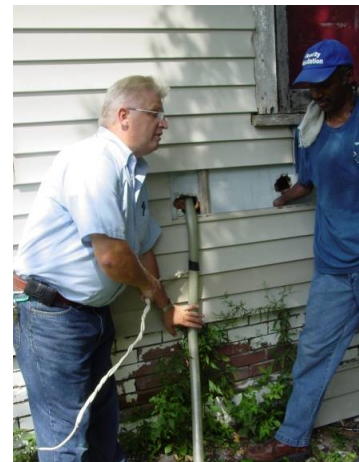
Figure 2142-1: Dense-pack cellulose being installed
