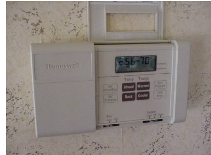
Figure 318-2: Automatic setback thermostat
