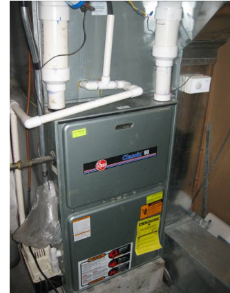
Figure 3133-1: Direct vent sealed combustion furnace
