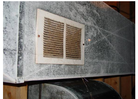
Figure 31531-4: Permanently seal registers in unconditioned spaces
