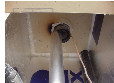
Figure 31111-3: Ensure that vent is properly connected
