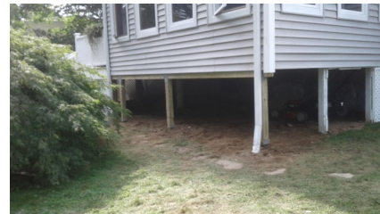
Figure 2154-1: Crawl space supported on piers
