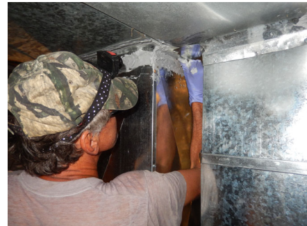
Figure 3124-1: Repair duct system
