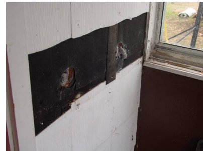
Figure 2141-1: Asbestos siding that has been removed
