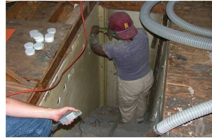
Figure 2135-3: Stairwell walls being dense-packed
