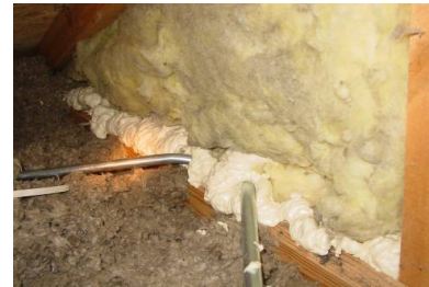
Figure 2122-3: Stud cavity sealed with 2-part spray foam
