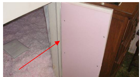
Figure 21365-1: Knee wall hatch insulated and weatherstripped
