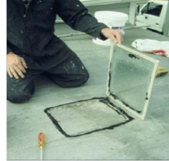
Figure 41612-2: Patch hole with galvanized steel and roof cement
