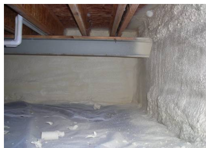
Figure 2151-2: Two-part spray foam applied to foundation wall with ground cover
