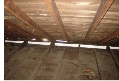
Figure 21324-1: Foam blocking installed over top plates
