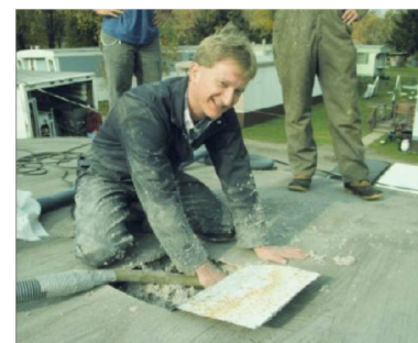
Figure 41612-1: Blowing insulation through mobile home roof
