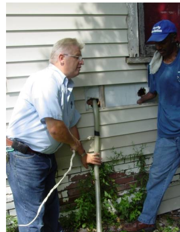
Figure 2142-1: Dense-pack cellulose being installed
