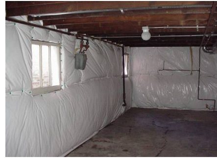
Figure 2162-1: Vinyl faced fiberglass insulation
