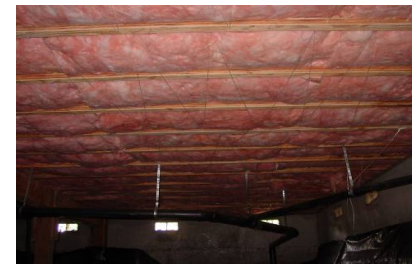
Figure 2152-2: Twine used to hold batt insulation in floor above crawl space
