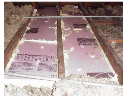
Figure 2122-2: Soffit sealed with foam board and 2-part spray foam
