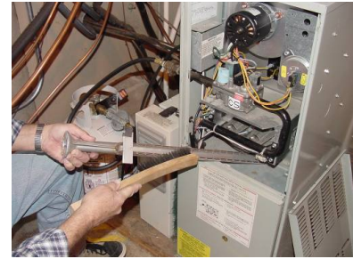
Figure 31111-2: Clean burners with stiff brush
