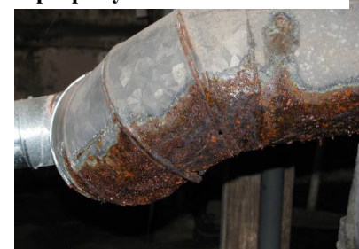
Figure 31111-4: Check vent for condensation problems
