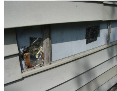
Figure 2142-2: Hole sealed with sheathing tape
