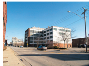
Vacant industrial building
