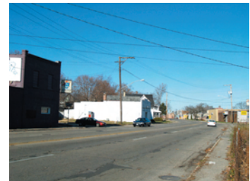
Typical roadway conditions on the north include potholes and broken sidewalks.
