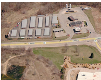
The storage facility has a large unscreened paved area fronting South Main (Source: Google Images).
