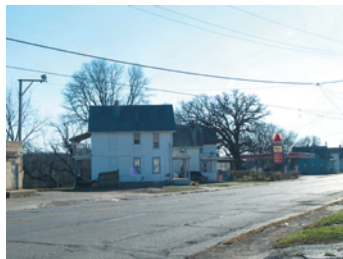
Residences on the east between Lincoln and Michigan Avenues
