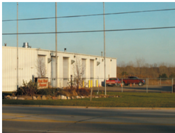
A chain link fence surrounds Rock River Disposal's property, which detracts from its appearance.
