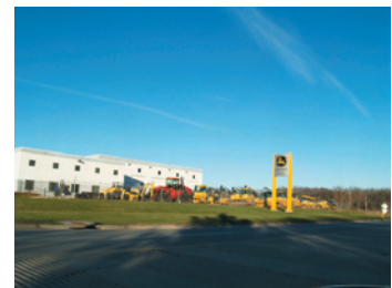
The tractor sales display area lacks screening.
