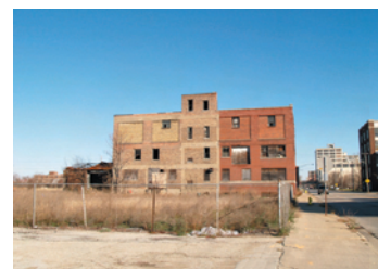
Current conditions at the rail yard site (both images above).
