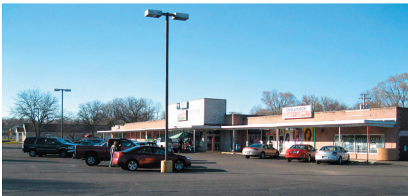
Strip center development on Marchesano Drive and South Main Street
