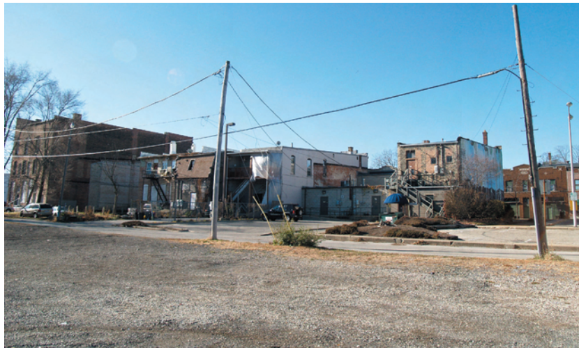
The existing alley and service areas for many buildings are not well maintained.
