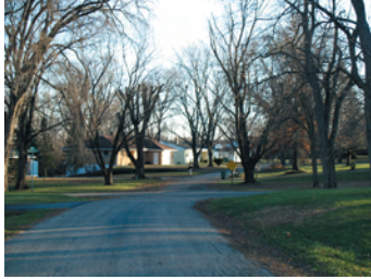
The older residential neighborhood in Zone C lacks curbs, gutters and sidewalks.
