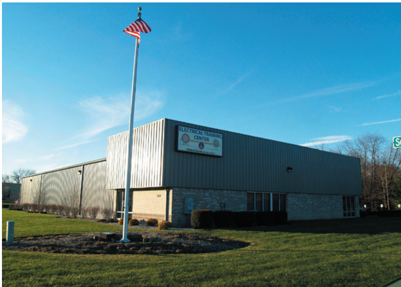
Southrock Industrial Park has a low vacancy rate and is an important employment center.
